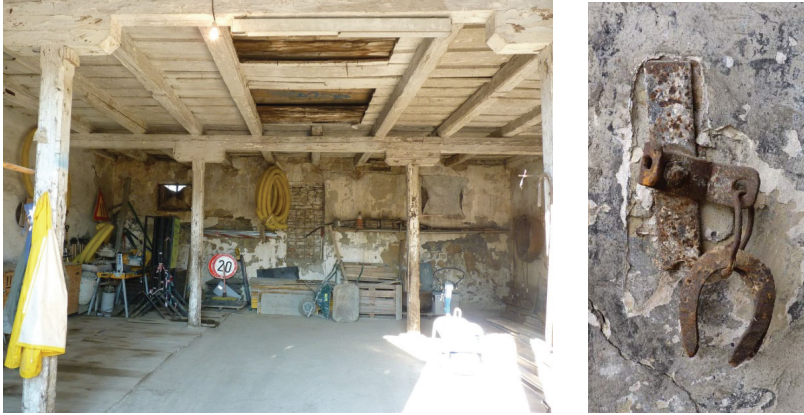
Figure 7 The stall interior with the preserved details
