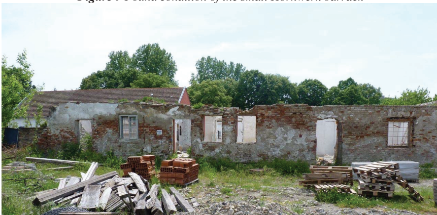
Figure 9 Found condition of the small Hornwerk barrack
