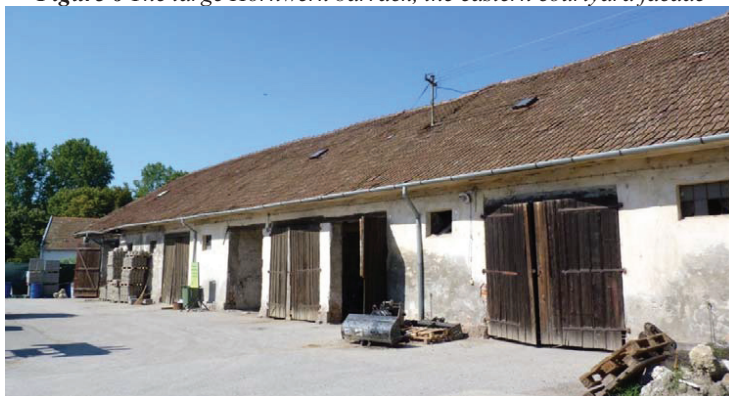
Figure 6 The large Hornwerk barrack, the eastern courtyard facade
