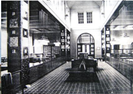
Picture 21 Forgotten central hall of Savings Bank
