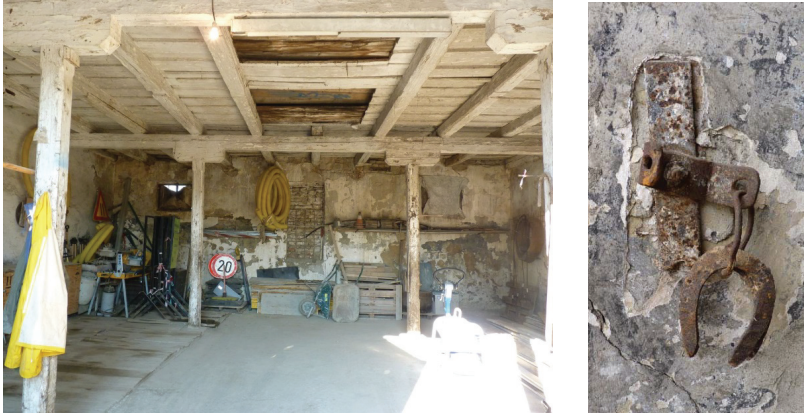
Figure 7 The stall interior with the preserved details
